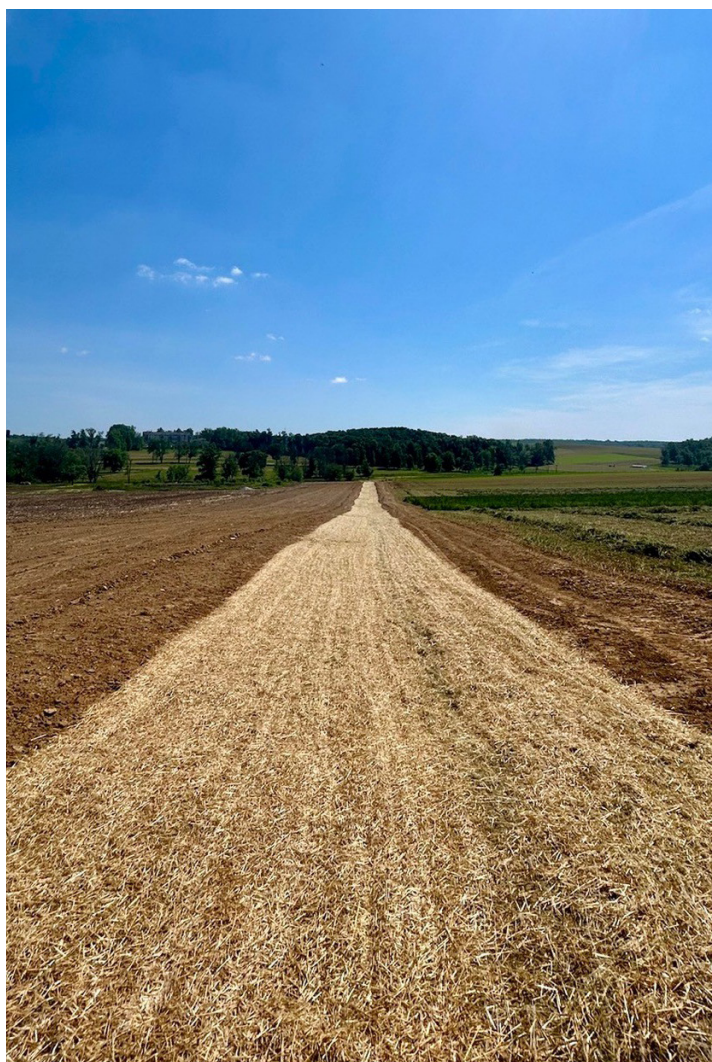
A grass waterway are channels lined with vegetation to convey water runoff without causing soil erosion and protect water quality.
