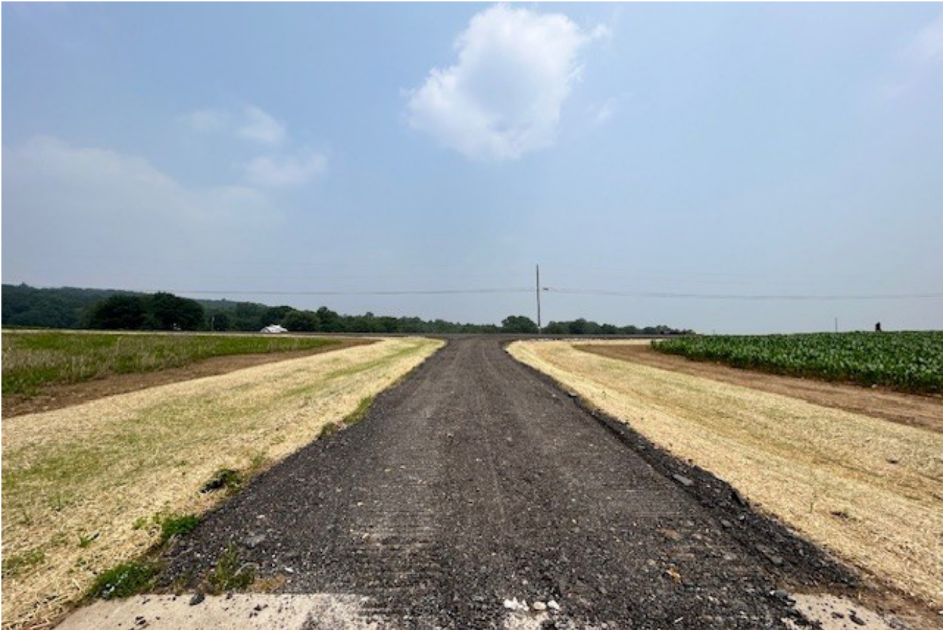
Swales are shallow channels with gently sloping sides that are used to manage stormwater runoff. Here they can be seen along either side of the drive.
