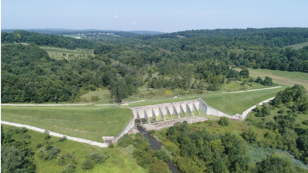
Barneston Dam in Wallace Township on the East Branch Brandywine Creek is a dry dam with a standard weir control on the auxiliary spillway
