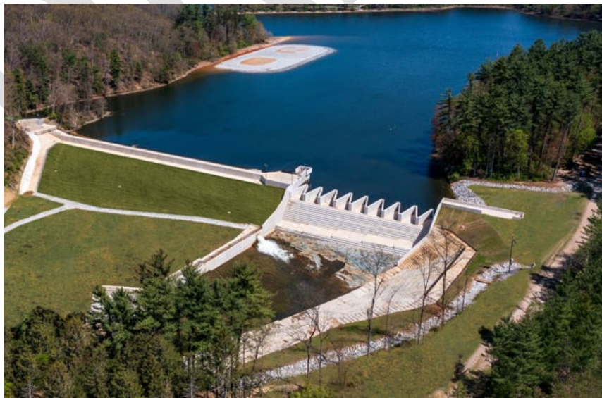
A labyrinth weir constructed at Lake Williams Dam in York, PA (photo courtesy of Gannett Fleming)
