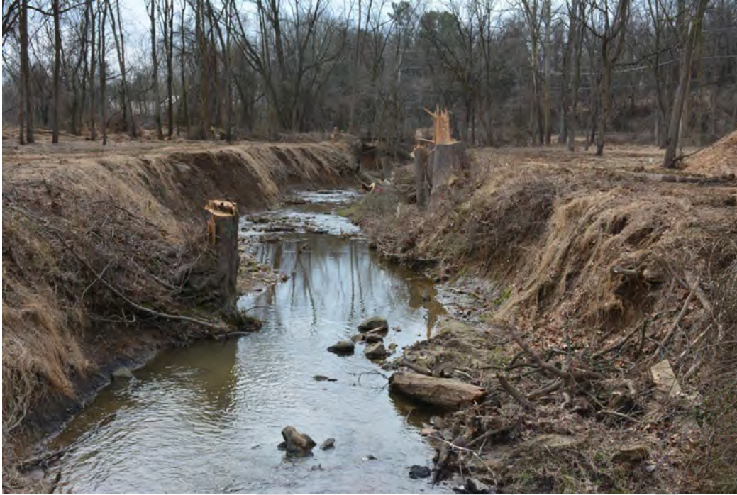
Plum Run in the lower Brandywine Creek watershed prior to restoration (photo courtesy of the Brandywine Red Clay Alliance)
