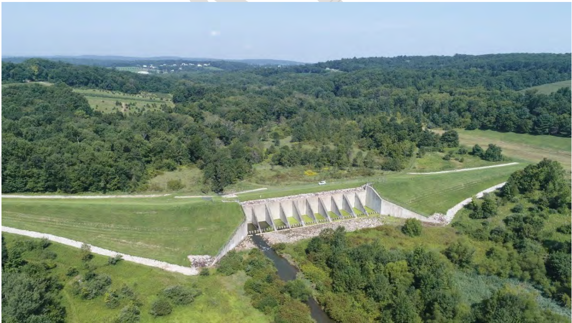
Barneston Dam in Wallace Township on the East Branch Brandywine Creek is a dry dam with a standard weir control on the auxiliary spillway, August 10, 2018.
