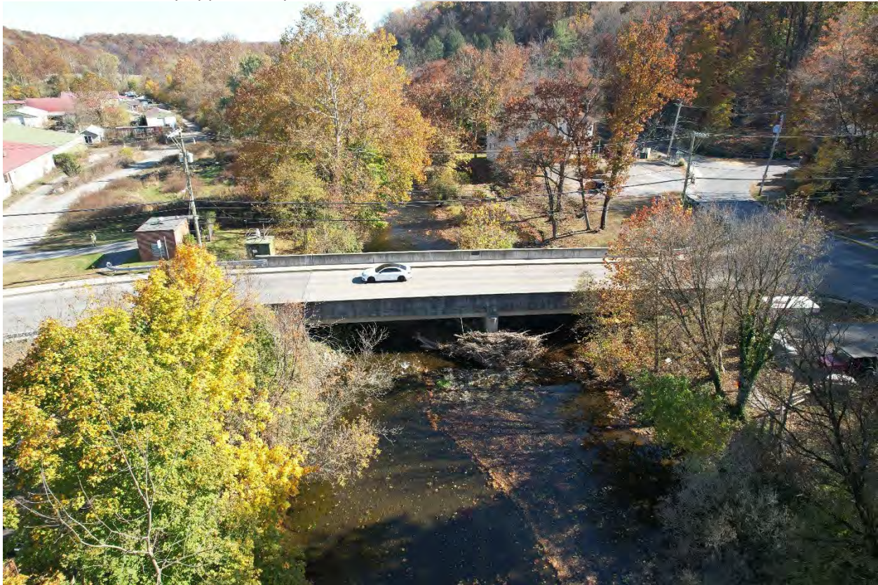
Union Street Bridge over the West Branch Brandywine Creek in Modena Borough, October 31, 2024.
