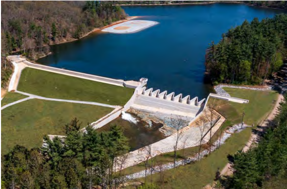
A labyrinth weir constructed at Lake Williams Dam in York, PA. Photo courtesy of Gannett Fleming.
