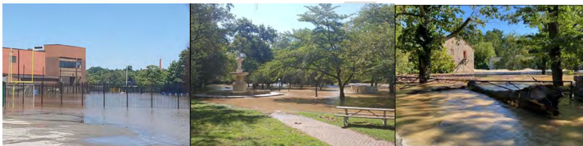
Figure 2.5 Hurricane Ida high water mark at Howard High School, the Josephine Fountain, and Brecks Mill (Dam No. 7) on the Brandywine in Wilmington, Del.
