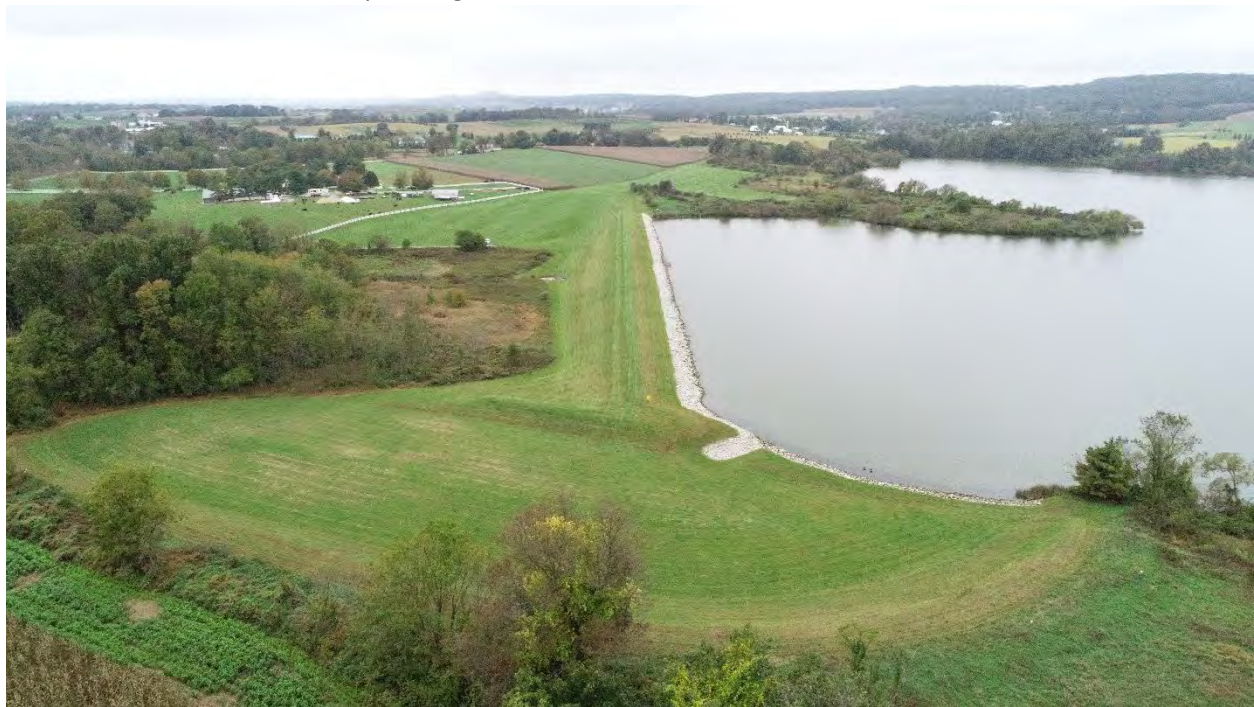
Struble Lake and Dam in Chester County, PA
